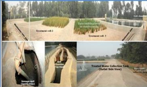
Community Scale Urban Wastewater Treatment Facility for augmenting irrigation water supplies at IARI experimental farm
