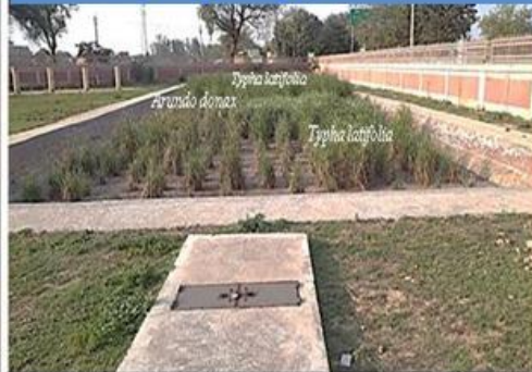
Community Scale Rural High SAR-Saline Sewage Treatment Facility at Pandit Deen Dayal Upadhyay Village, Mathura, UP
